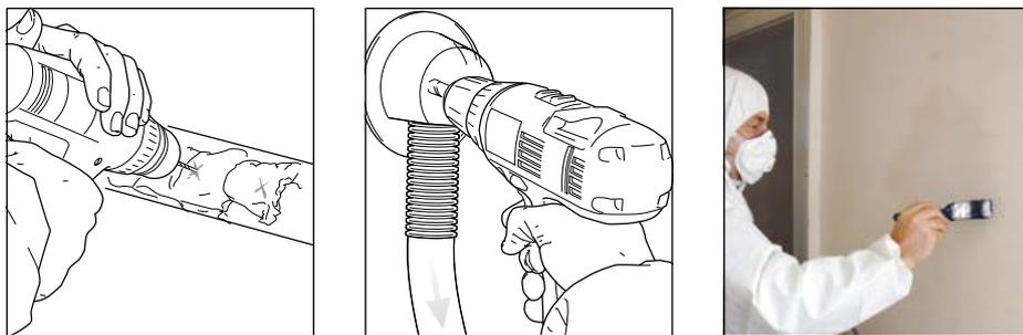
Drill through masking tape covered with paste or foam, or use a drill cowl connected to a Class H vacuum cleaner as local extraction. Seal drilled edges with sealant
